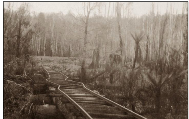
Fire-buckled rails on the Loch Valley Tramway north of Noojee after the 1926 fires.
