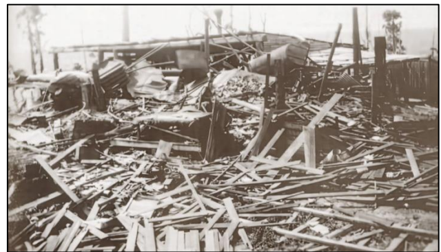
Marchbank's mill in February 1937, soon after the winch boiler had exploded. Photo: Jack Haigh.
