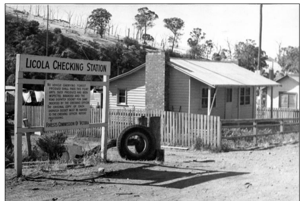
Licola Checking Station.
