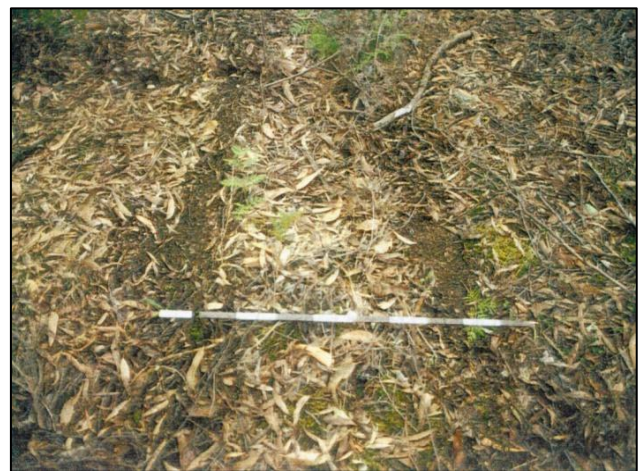
The surviving tramway formation is approximately 2 metres across and raised 300mm above the surface of the ground on either side. Distinct sleeper impressions spaced about 900mm apart can be discerned along much of the surviving formation, which includes a gentle curve at the northern extremity. The condition of the surviving remains is remarkable given their great age. Photo by Peter Evans.
