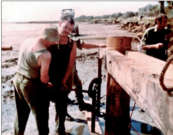
Erecting jetty piers. Photo used with permission from the RAE Association: https://raevictoria.com
