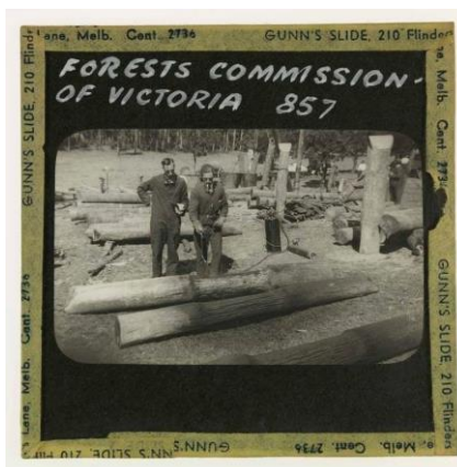
Oxy-acetylene treatment of poles. Pole test site, Glen Park, 1936.
