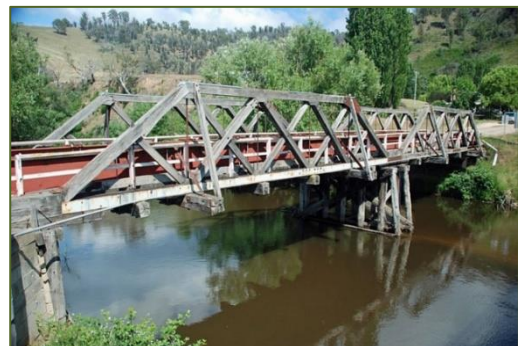
The Hinnomunjie truss bridge – the only timber truss bridge remaining in Victoria. Photo credit: Victorian Heritage Database.
