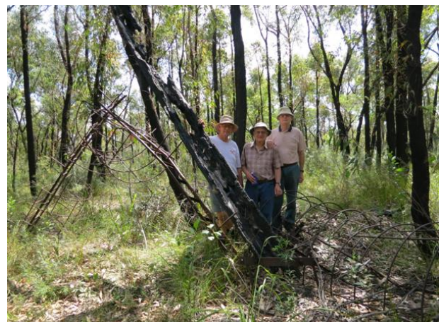
Figure 2: Remains of Woodburn Fire Tower 30 October 2012 showing the single pole, ladder, basal collar and safety mesh. Observers left to right - Ian Barnes, Len Mors and Ian Bevege.
