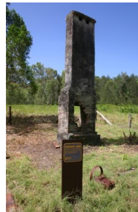
Chimney from the 20th century farmhouse, constructed from mill period bricks (Photo: MPAP).
