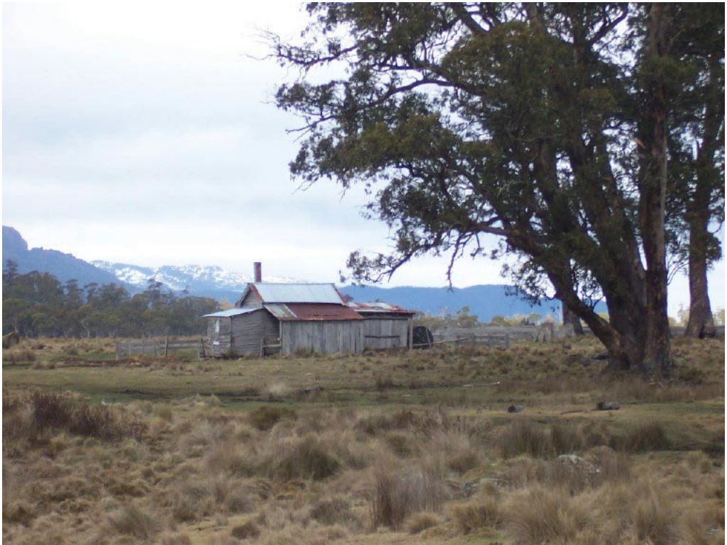
Figure 3. The historic Borradaile Hut (Author's photograph).
